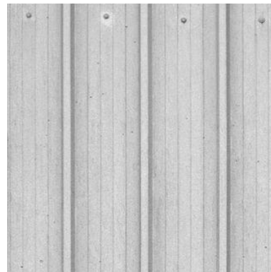
GALVANIZED STEEL CLADDING
